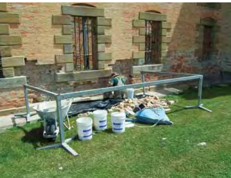
Conservation work at Port Arthur.
