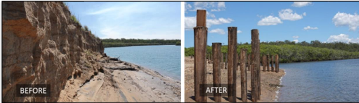
Photo: Example of a before and after photo of a riverbank that has been stabilised to reduce future sediment and run-off reaching the Reef.
