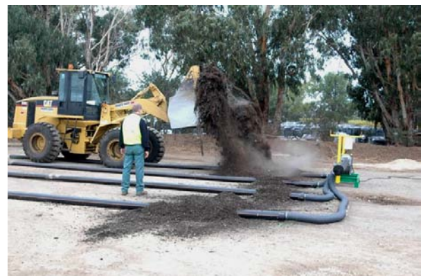
Establishing a mobile aerated floor (MAF) composting pile
